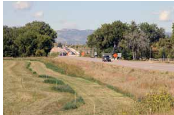
Widening of Harmony Road near I-25 in Timnath
