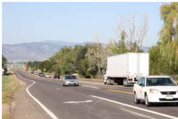
SH 14 near I- 25 in Larimer County
