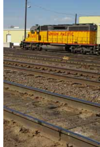
Union Pacific Railroad switching station in LaSalle
