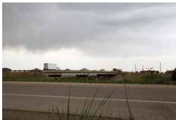
The SH 392 bridge over I-25 in Windsor
