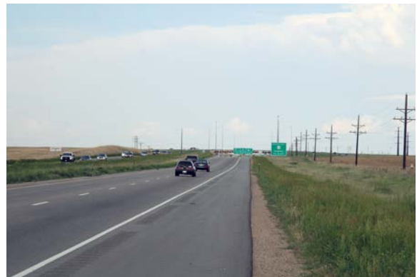
Looking East on US Highway 34 just outside of Greeley
