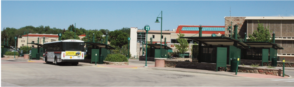
Lory Transit Center, image courtesy of the CSU Facilities Management website
