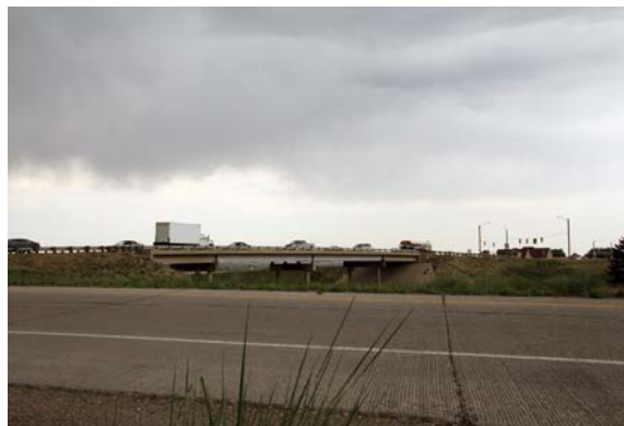
The SH 392 bridge over I-25 in Windsor
