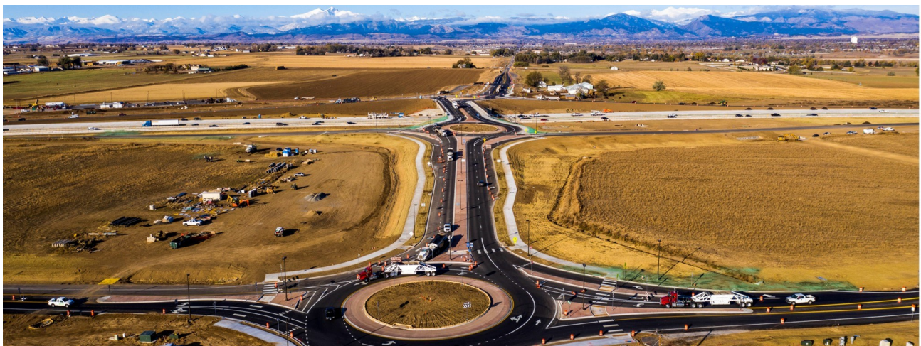
SH402 roundabouts under construction. Source: CDOT
