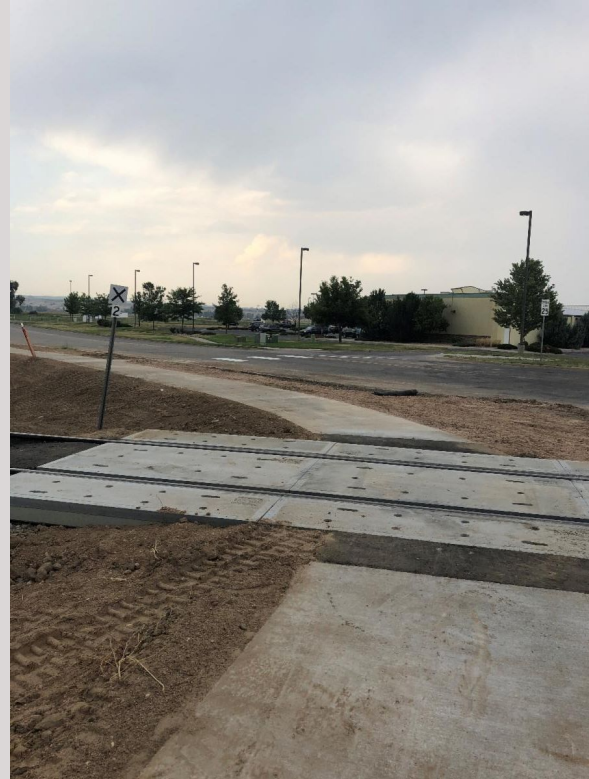
New sidewalks at UPRR crossings at Alice Street in Milliken.
