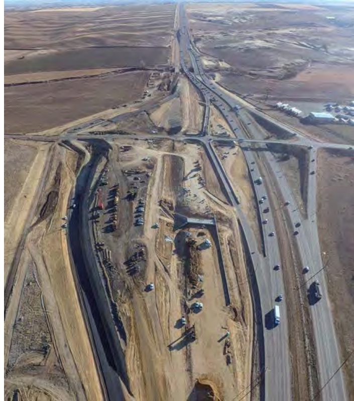
Aerial of SH 56 Realignment
