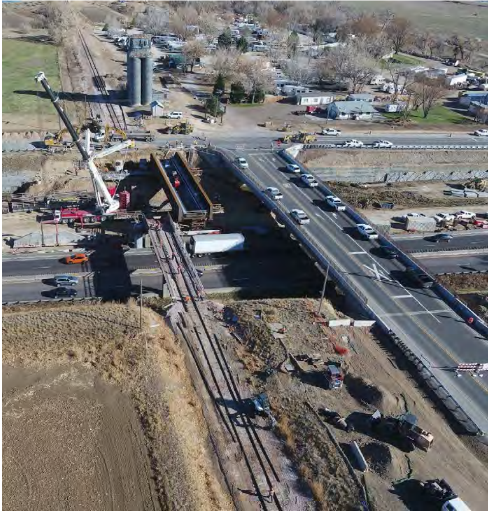
GWRR Slide-In Bridge (left) LCR 20E Bridge (right)
