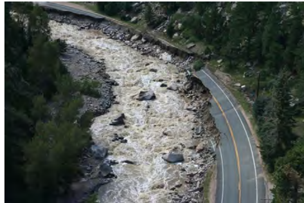
The images above show the immediate aftermath (left) of the 2013 floods on US34 in Big Thompson, as well as the recovery and mitigation efforts to realign the roadway out of the floodway (right). The reconstruction was named Best of the Best out of 820 construction projects nationwide by Engineering New Record. (Image credit: CDOT)
