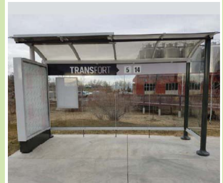
Upgraded Bus Stop—Transfort
