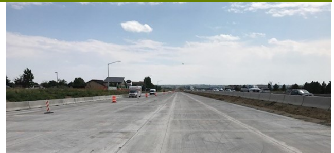
I-25 roadway near Crossroads. Image Credit: CDOT
