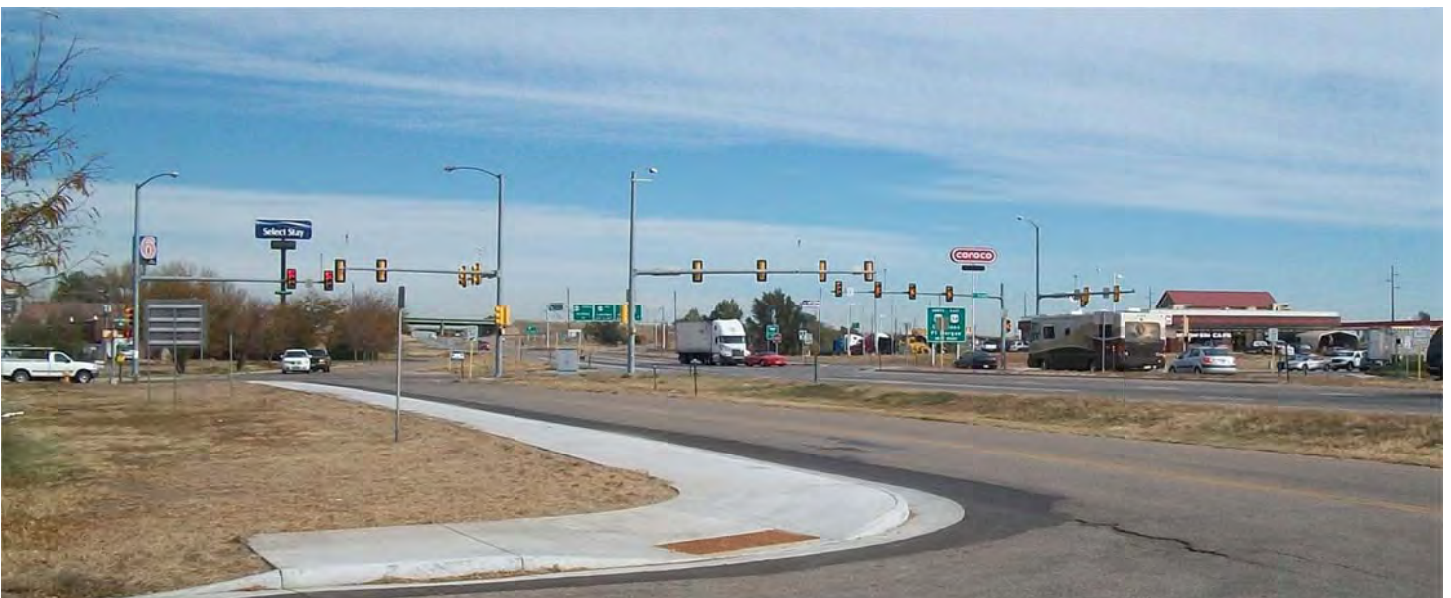
Existing Intersection Looking Northeast
