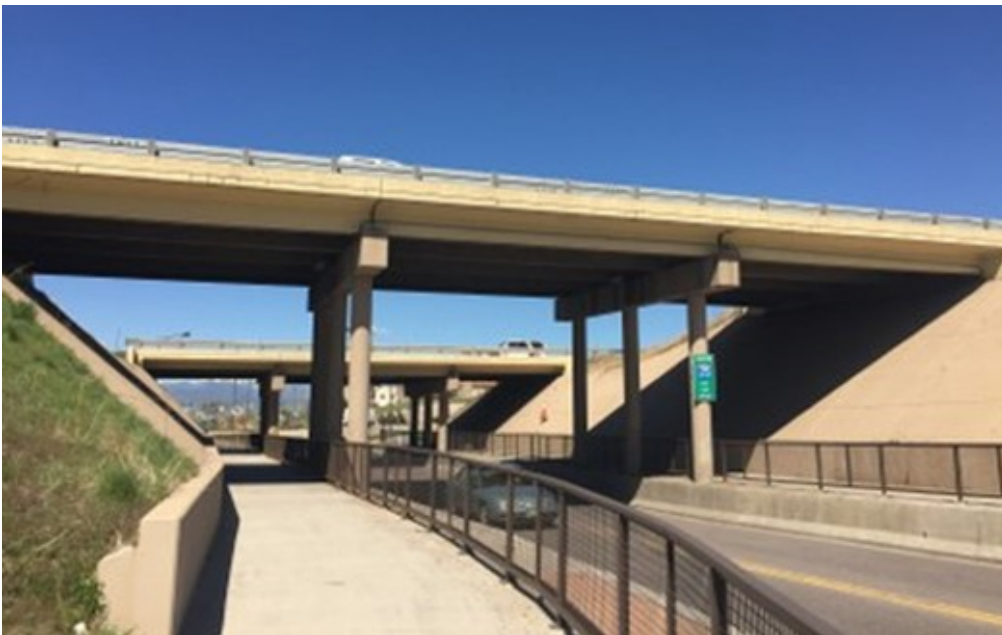
N I-25 Crossroads Bridges
