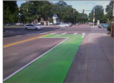
A Bike Box at W Plum St. & Shields St. in Fort Collins
