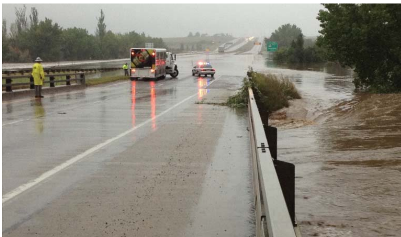
Figure 10. Morning of September 13 at 0716 hours. Looking south. Photo Credit: James Flohr, CDOT Resident Engineer.
