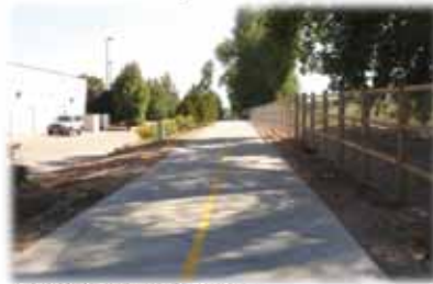
Parallel Path with Fencing
