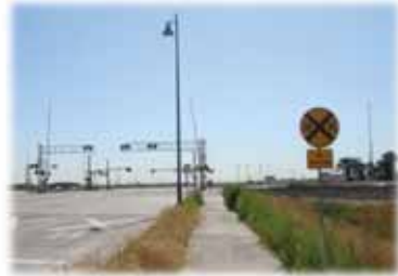
Path with At-Grade Road Crossing
