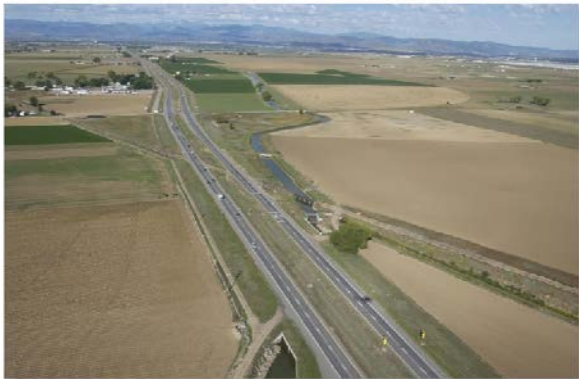
US 34 east of I-25 looking west. |
