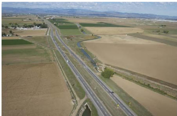
US 34 east of I-25 looking west.
