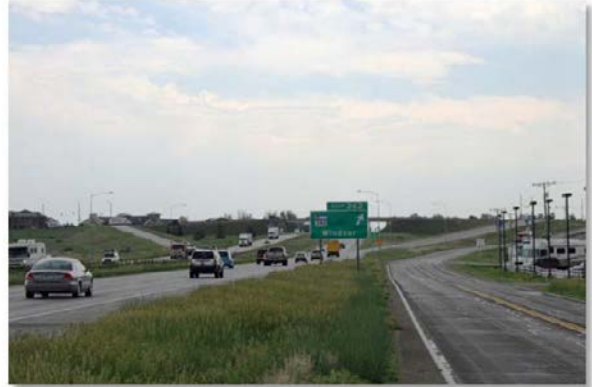
Southbound I-25 approaching the SH 392 interchange in Windsor.
