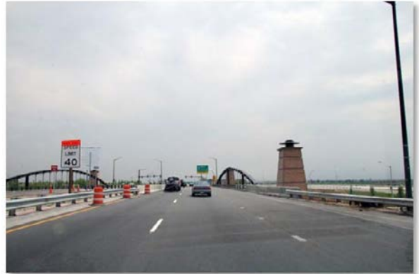
The I-25/US 34 interchange was recently reconstructed
