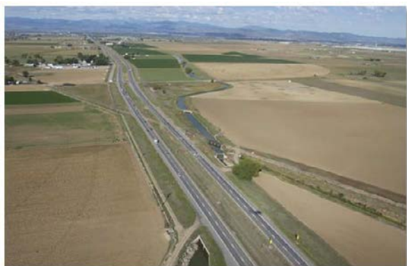
US 34 east of I-25 looking west.
